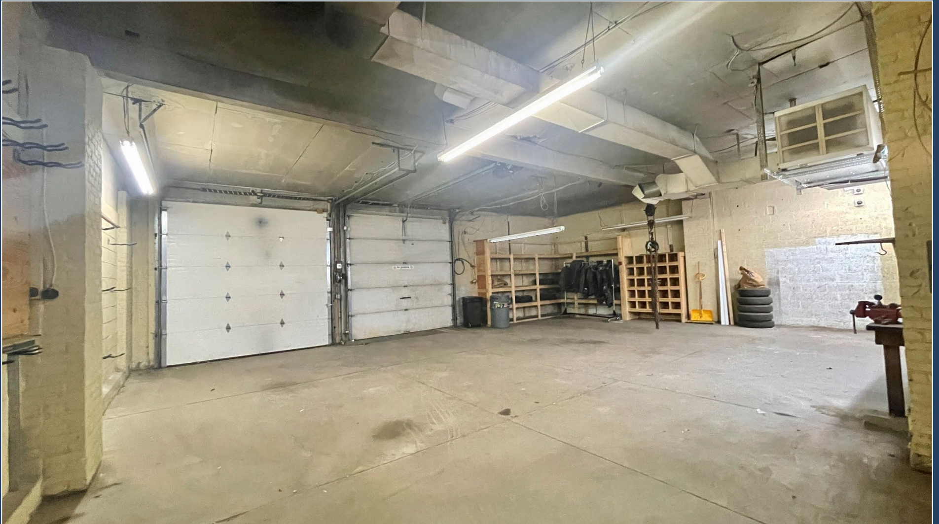
Garage with Four 10' H x 10' W Drive-in Doors
