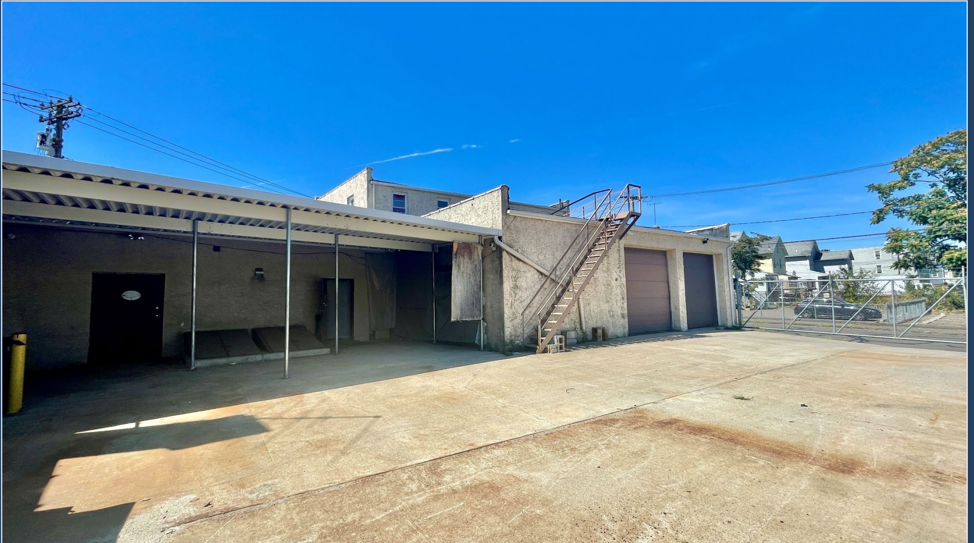
Gated Lot with Canopied Area in Rear of Building
